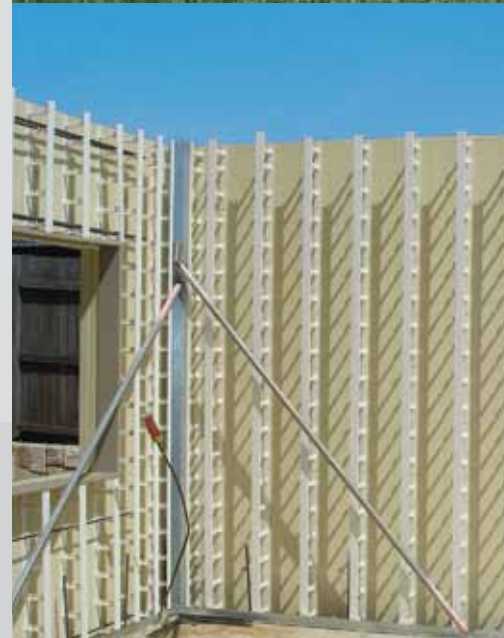
Wall 15 No Insulation External Polymer Cladding built-in Drainage Channels Internal Polymer Timber built-in Service Cavity (for carports)
